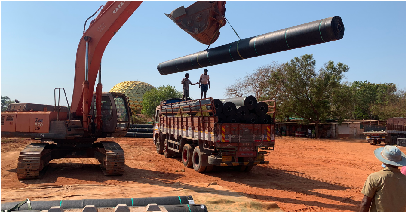
Rolls of HDPE waterproofing membrane being unloaded in early April 2026
