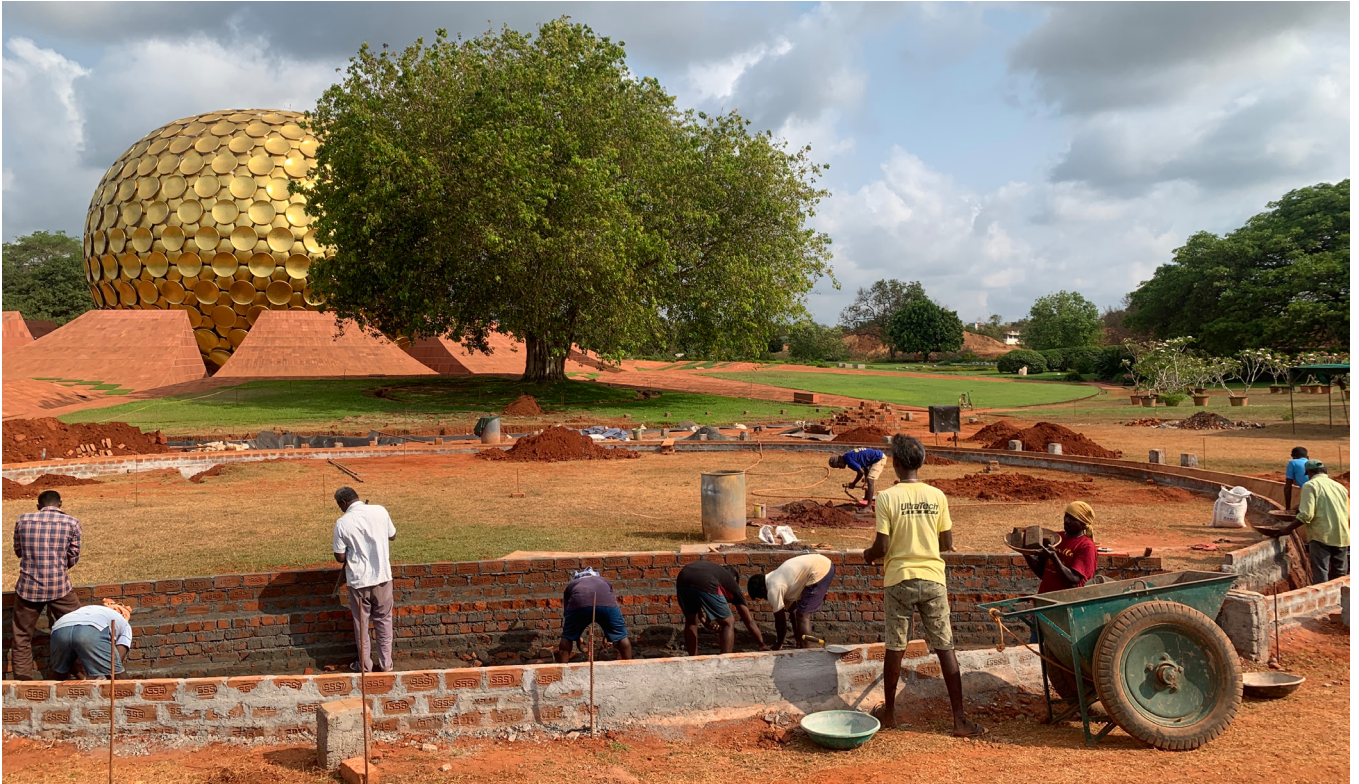
Construction work on the Garden of Harmony is well underway
