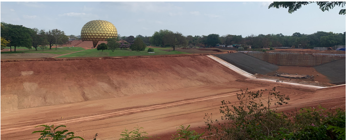
The three hundred meter long section two of the Matrimandir Lake is being prepared to receive its waterproofing layer
